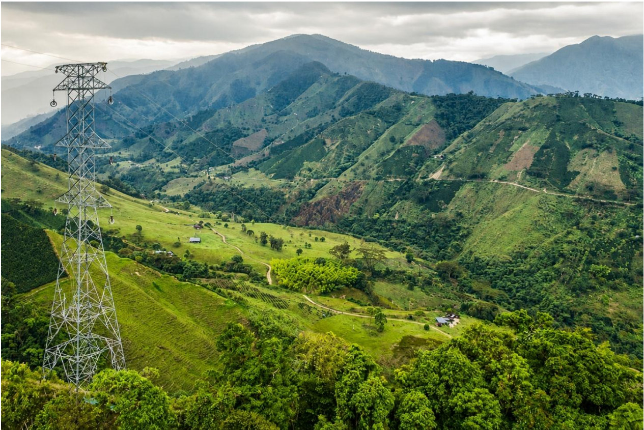
Figure 15 Electricity-transmission towers operated by Enlaza (Grupo Energía Bogotá) in mountainous Colombian terrain (Tesalia–Alfárez 230 kV line). Source: Enlaza – Grupo Energía Bogotá.
