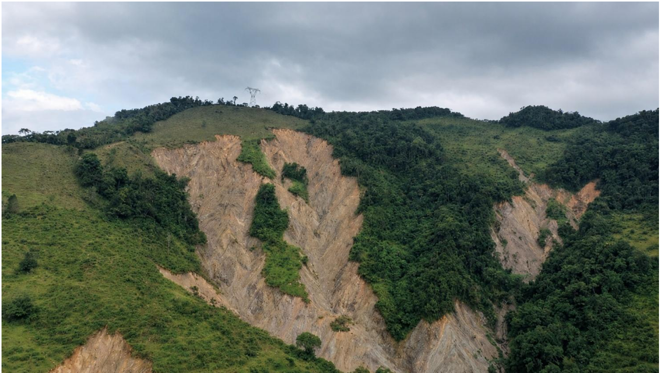
Figure 14 GeoAndina monitoring of the La Reforma transmission-line corridor. Source: Restrepo Botero & Piedrahita Ospino, Noticreto no. 170, pp. 38–41 (image courtesy of Geoandina i SAS).
