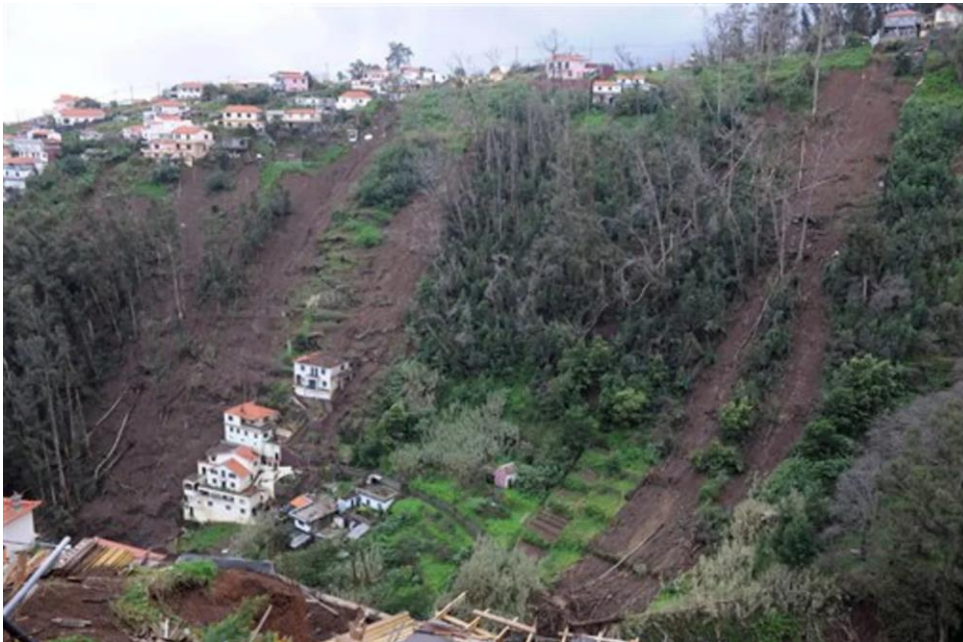
Figure 2-2: Landslide in Curral das Freiras, in Madeira, February 2010 17
