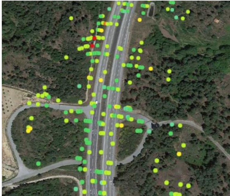
Figure 3-6: Part of the A24 with areas of severe subsidence represented by red dots
